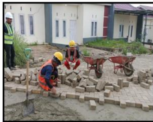
Gambar 10. Proses pemasangan paving block
